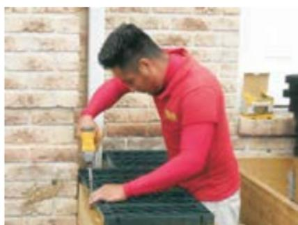
Fastens to floor joists with standard deck screws.
